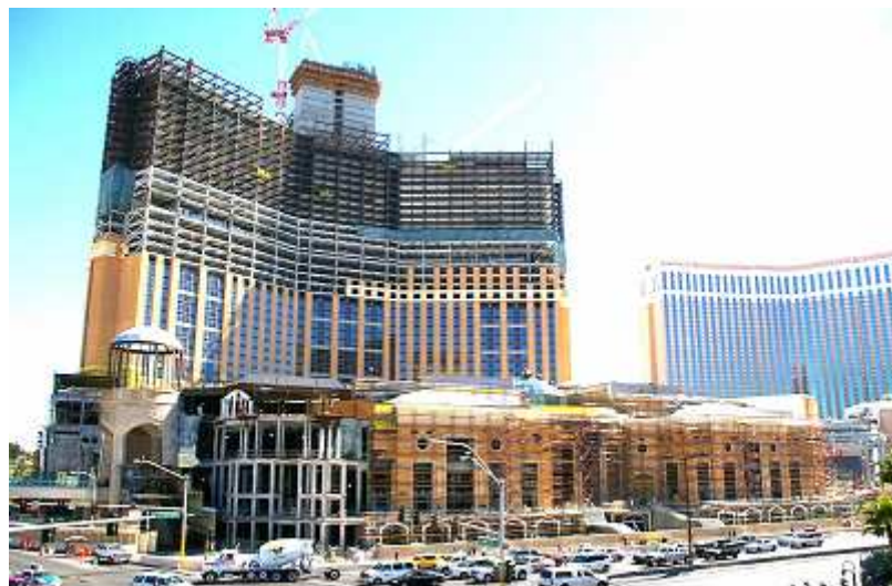
New casino in Las Vegas called "Palazzo" containing approximately 70,000t of structural steel. Detailed by BDS Steel Detailers – Brisbane
