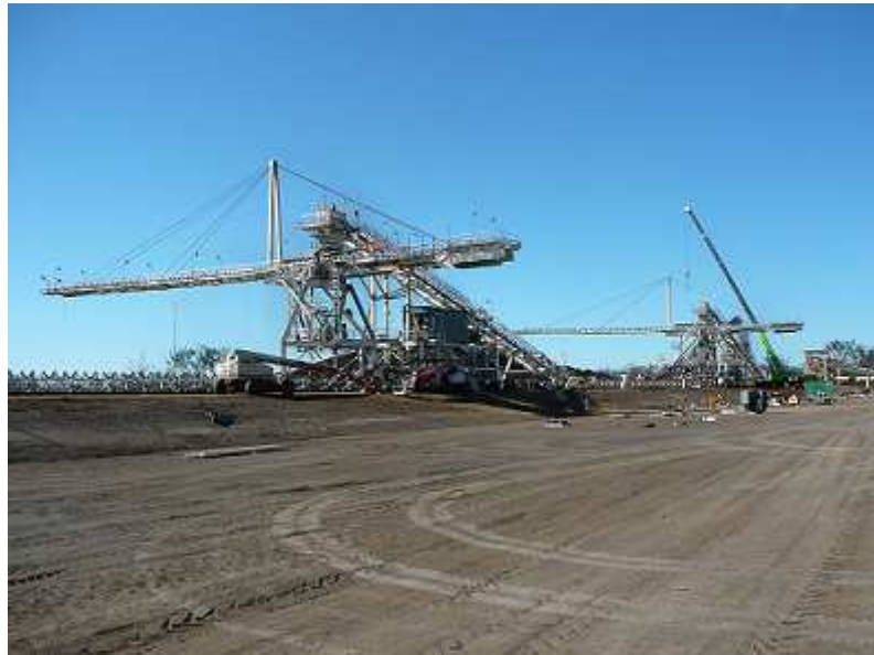
Two new coal stackers built last year at the Millennium Coal Mine, West of Mackay. Detailed by Steelcad Drafting Pty Ltd
