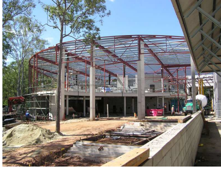
Steelwork as a Detailer sees it....
